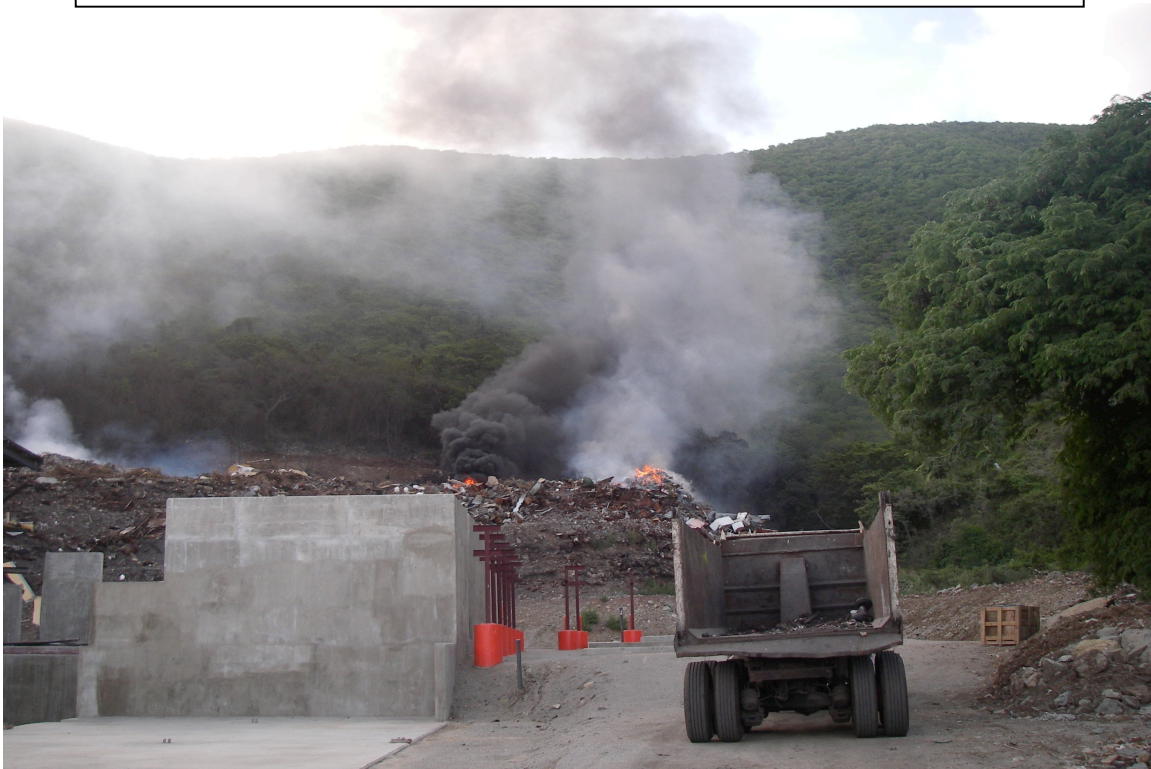
Smoke from burning dump behind incinerator during incinerator downtime
